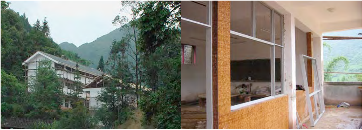
Pingbian (Yunnan) school under construction. Source: Tang Di
